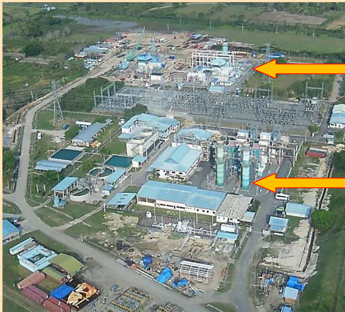
Aerial view of Sengkang Power Plant
