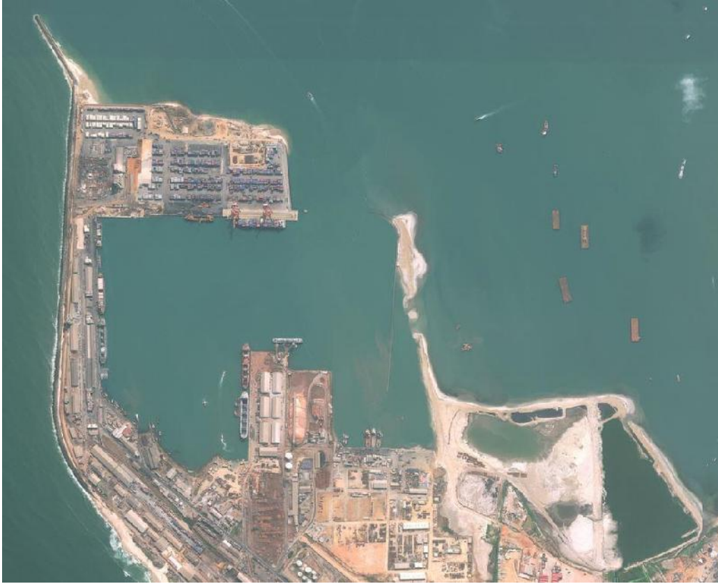
Figure 11: Aerial view of the port at Pointe-Noire showing new wharf progress
