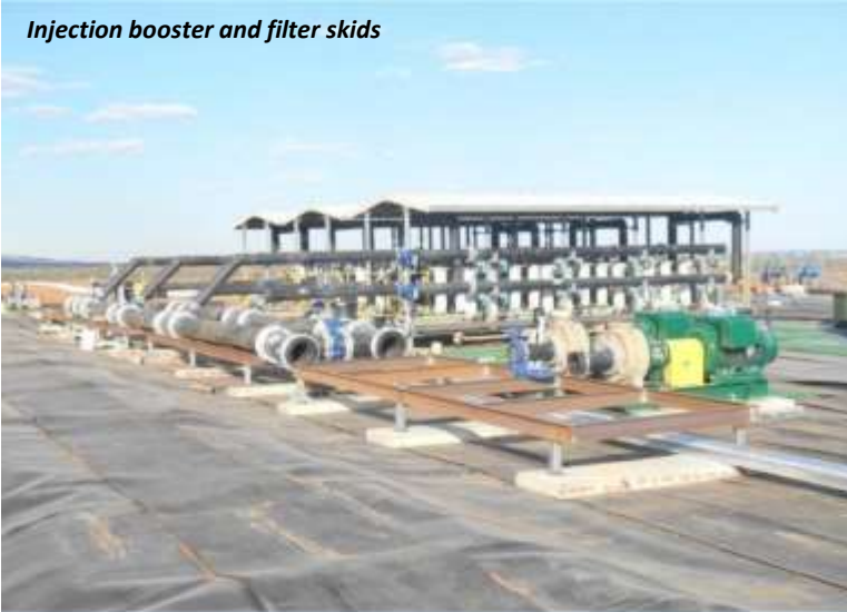
Installation of FME wellhouse 1 and filter skids
