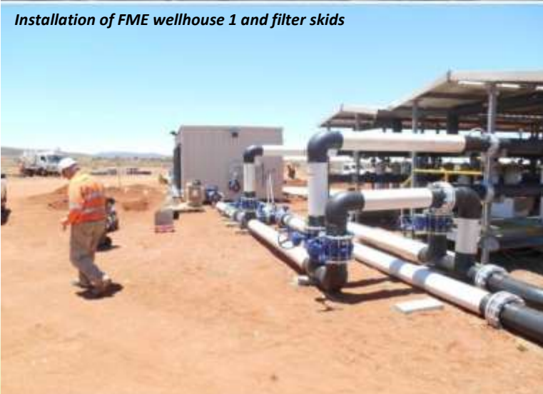
Lateral 'spiders' from wellhouse to FME wellfield
