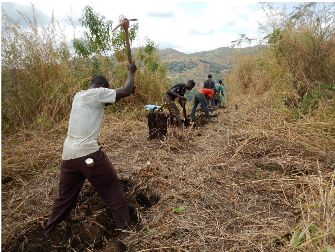
Photo 1. Clearing a trench line
