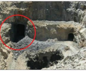
Figure 7-8: 490 stope breakthrough into open pit
