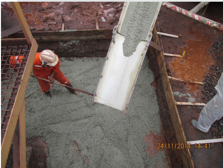
Figure 2; Pouring the concrete for the foundations of the tertiary crusher at Posse.
