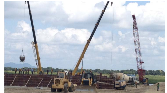
New Road and Bridge Constructions on route to Epanko
