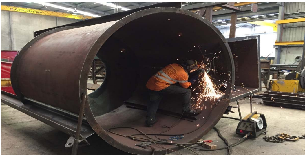
Beneficiation plant pump hoppers being fabricated in Perth
