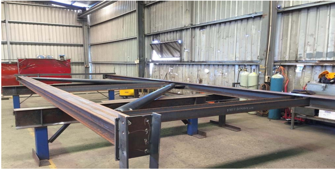
Structural module fabricated at workshop in Perth
