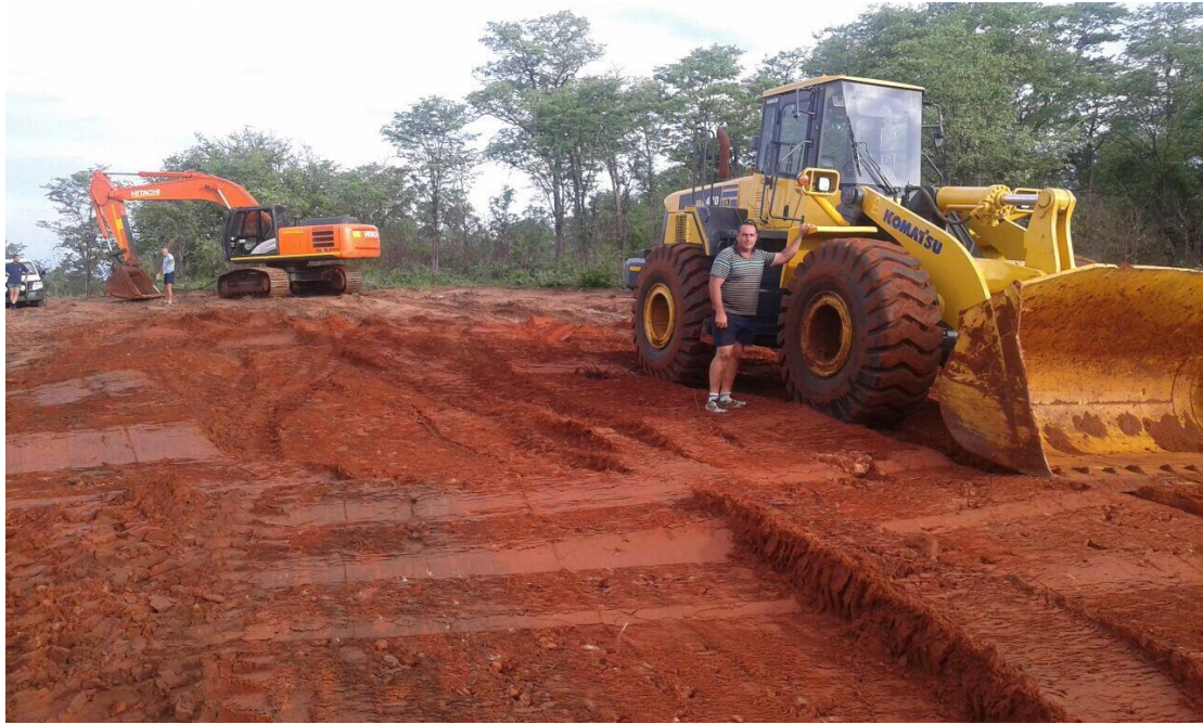
Clearing of site for the 100,000 tonne trial mining program
