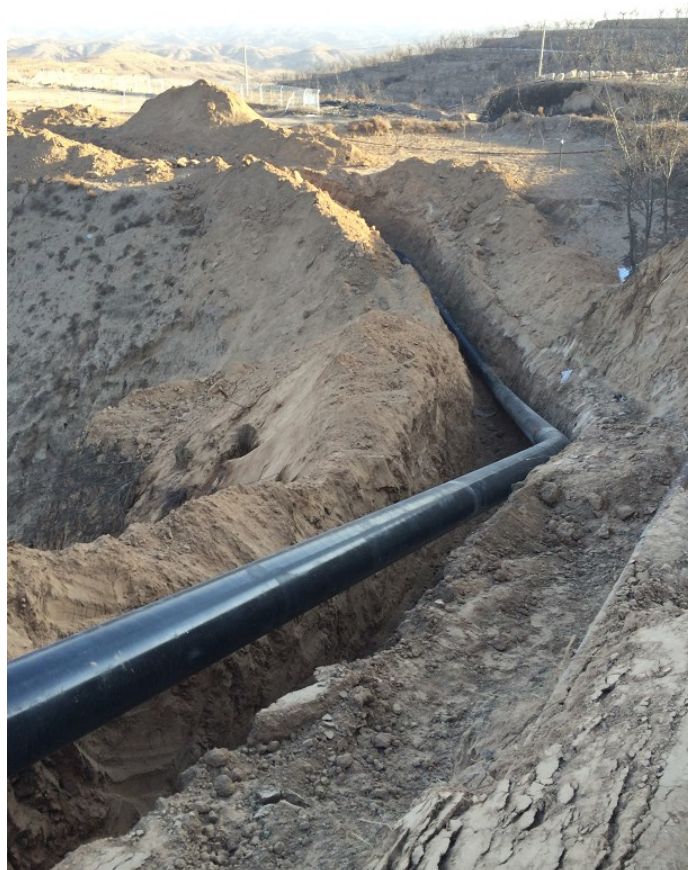
Laying of the third party spur pipeline and initial gathering lines on Linxing (West) is approaching completion.
