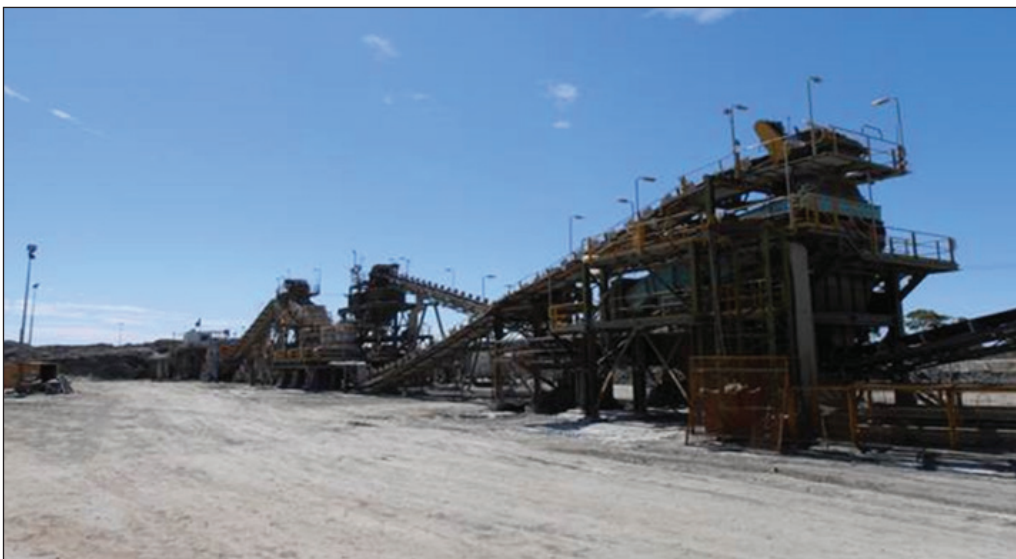
Figure 2: SIGM heap leach 3 stage crushing and screening plant (courtesy SIGM)
