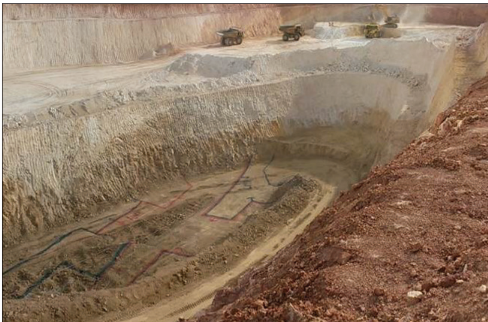
Figure 1: Stage 2 cut back progressing at the Kintore gold project
