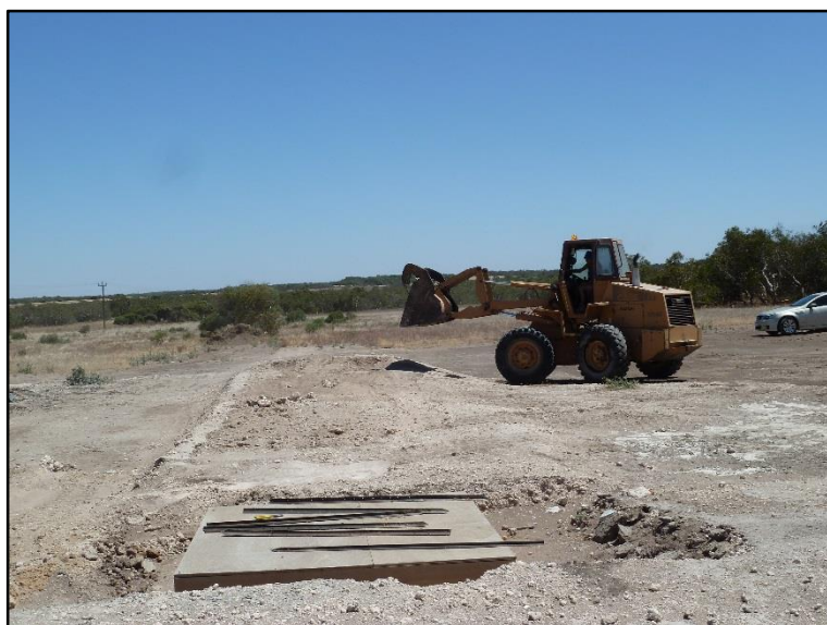
Key Services tidying up the ramp against the wellhead (box) in preparation for rig mobilisation
