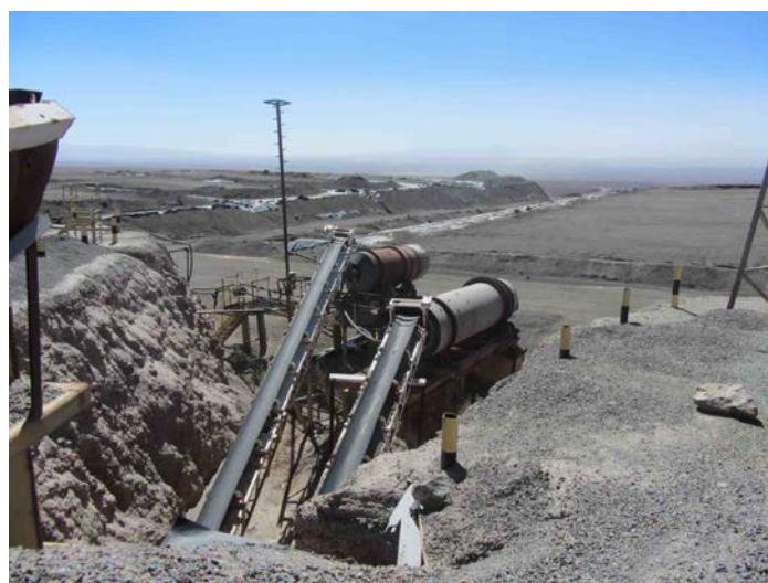
Figure 6 An abandoned copper oxide plant at Tuina
