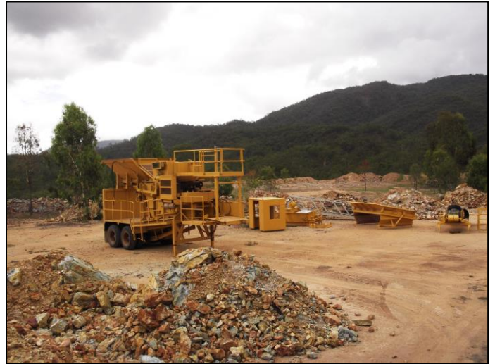
Picture 15: Primary crusher ready for final assembly.
