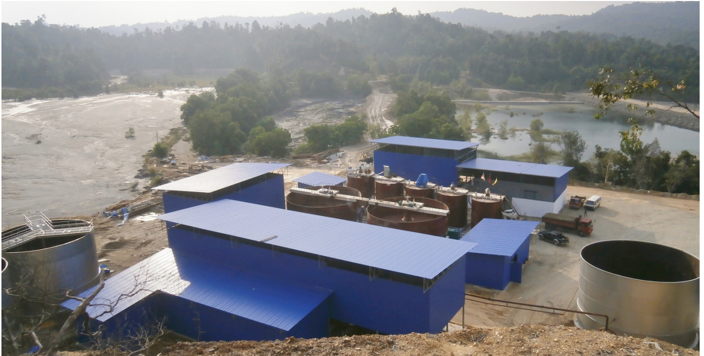
Photograph; Lubuk Mandi tailings treatment plant in foreground with existing tailings dam(back left) and new stage 1 waste storage facility (back right). Taken 5 November 2014.
