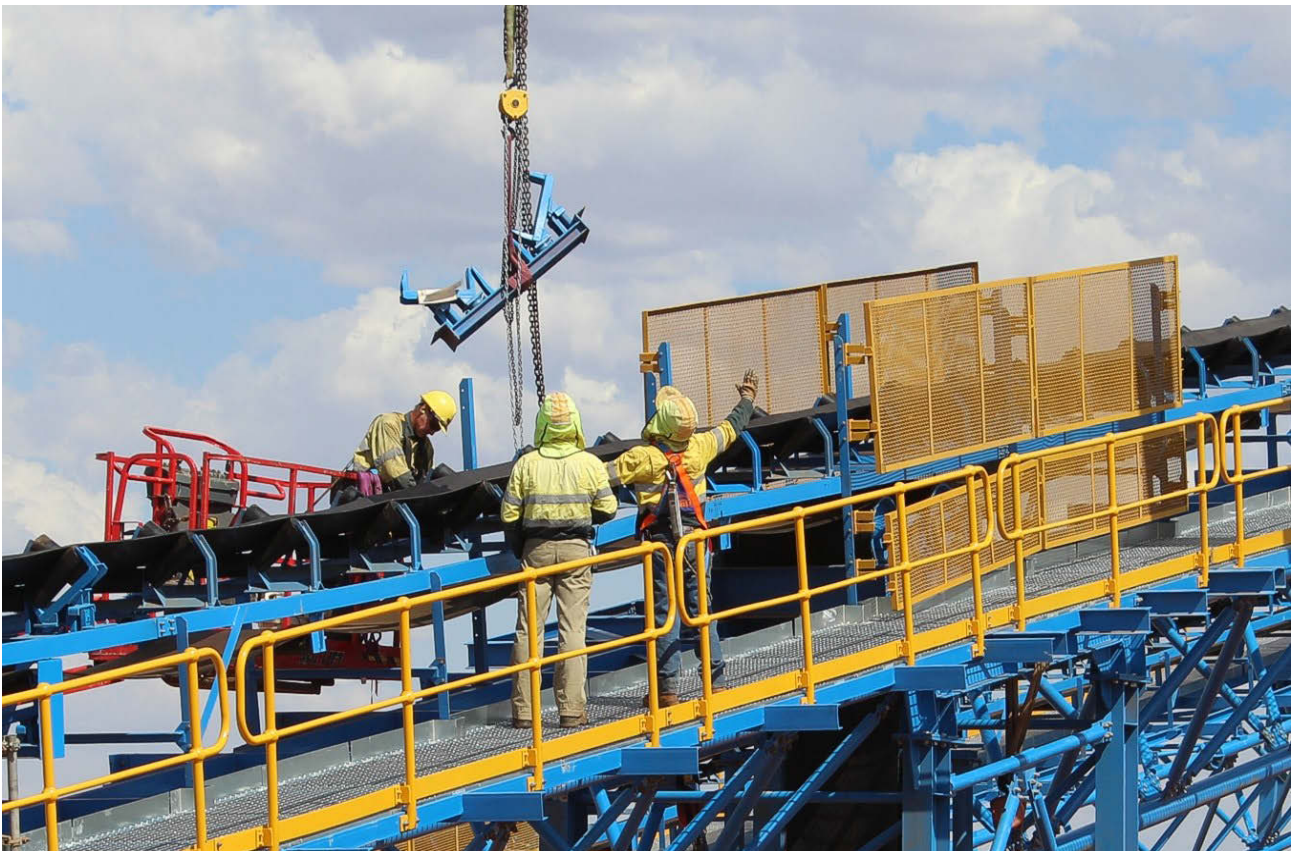
Figure 17: Rocklands Process Plant - major components installed, structural completion underway.
