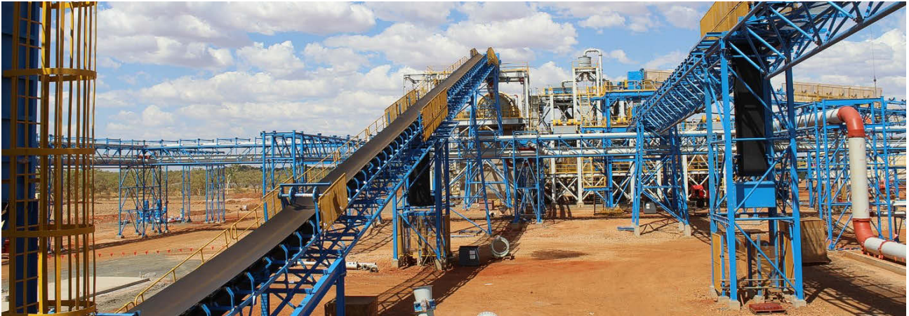
Figure 14: Rocklands Process Plant - major components installed, structural completion underway.
