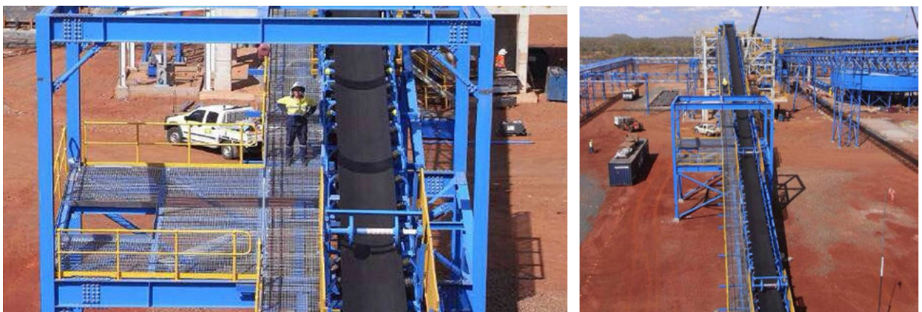
Figure 15: Rocklands Process Plant - major components installed, structural completion underway.
