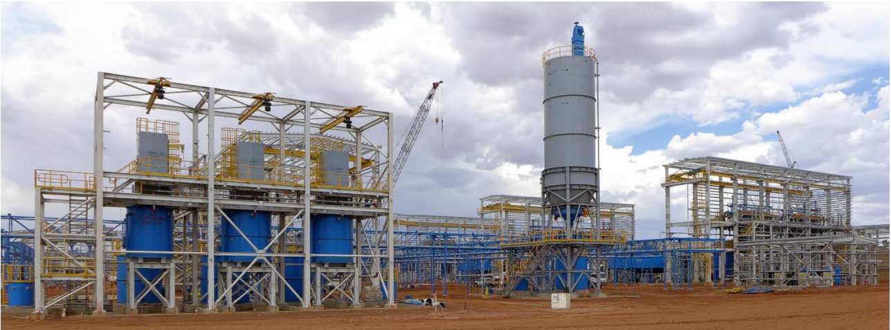
Figure 18: Rocklands Process Plant - major components installed, structural completion underway.
