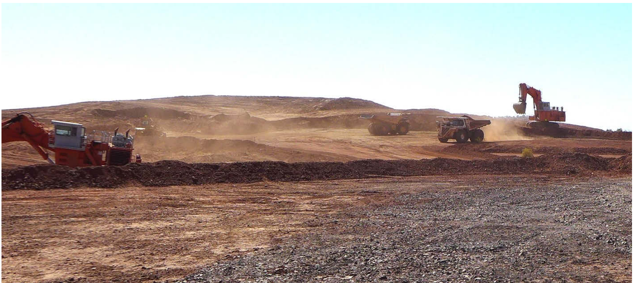
Figure 35: Mining at Rocklands South Pit commenced in free-dig areas. Middle image shows excavations at the base of Telstra Hill, looking to the north-east from the Rocklands South Pit. Bottom image shows the same scene looking to the east. The ROM and Process Plant can be seen in the far distance from the left of the image.
