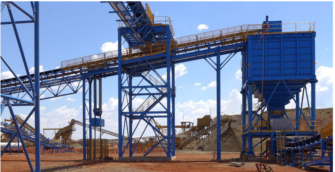
Figure 16: Rocklands Process Plant - major components installed, structural completion underway.
