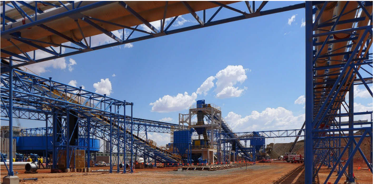
Figure 19: Rocklands Process Plant - major components installed, structural completion underway.
