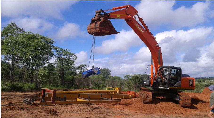
Deployment of Trial Mining Program equipment and preparation of site
