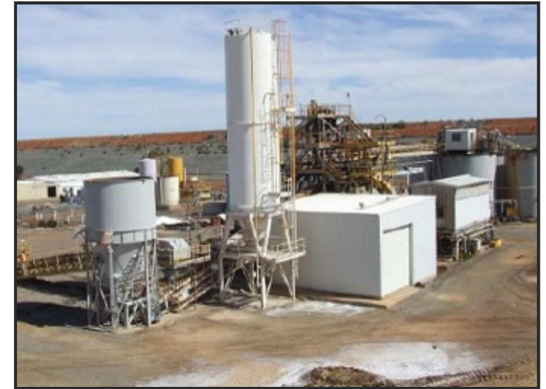
Kundana CIP Plant prior to decommissioning & refurbishment
