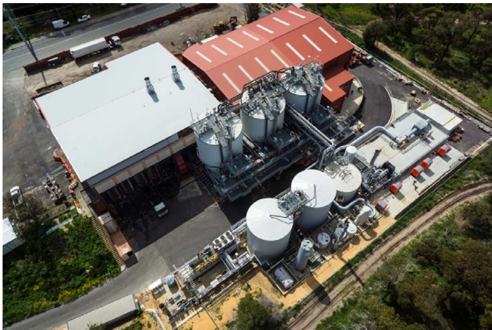
Figure 1: AnaeCo™ AWT Plant at WMRC JFR McGeough Resource Recovery Facility, Shenton Park, Western Australia
