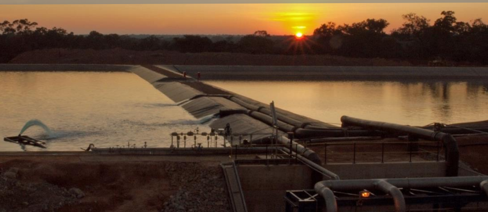
Pregnant liquor pond containing high grade copper in solution feed for SXEW
