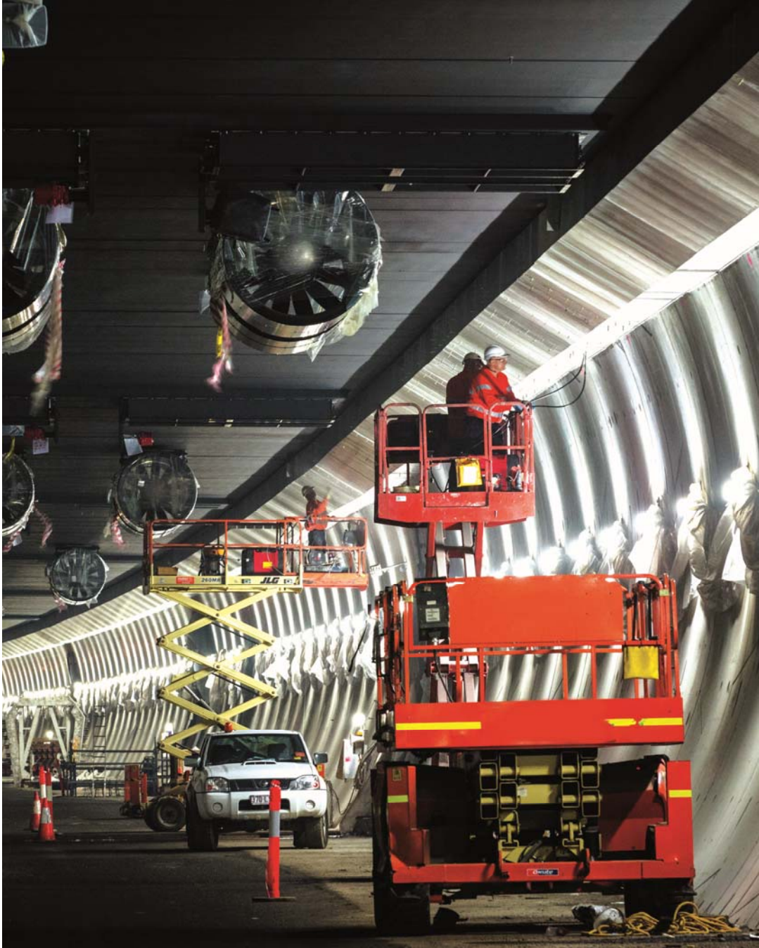
Ventilation fan installation at the Legacy Way Tunnel, Brisbane, QLD
