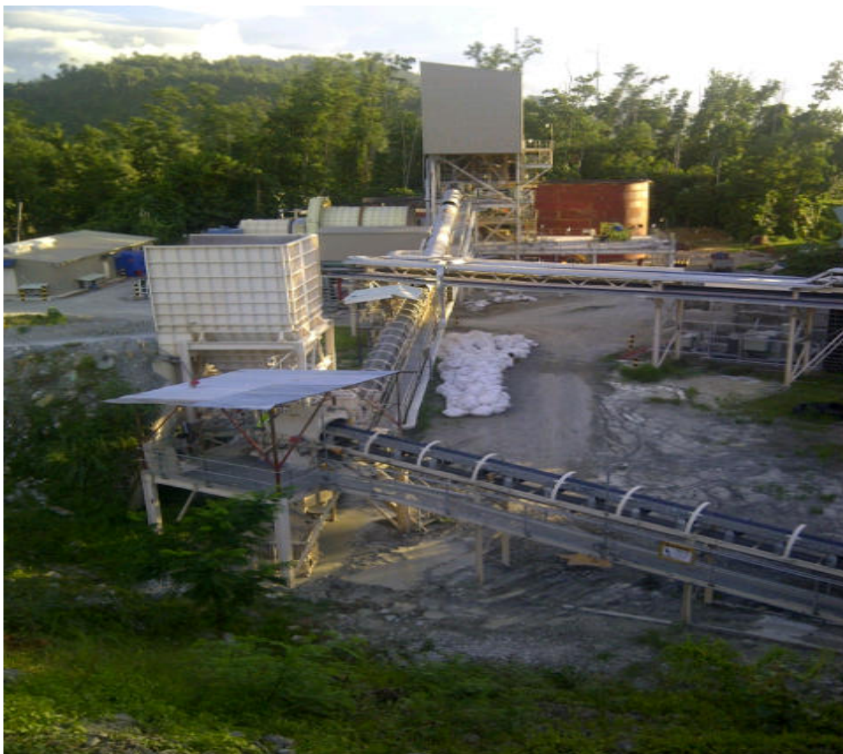
Photo 2. Mill site showing new leach tanks located behind the SAG mill.
