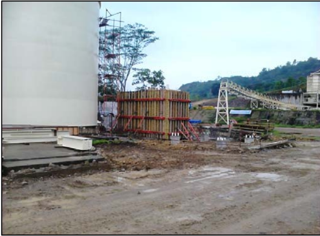
Figure 2 Existing MMC foundation and Gravity area
