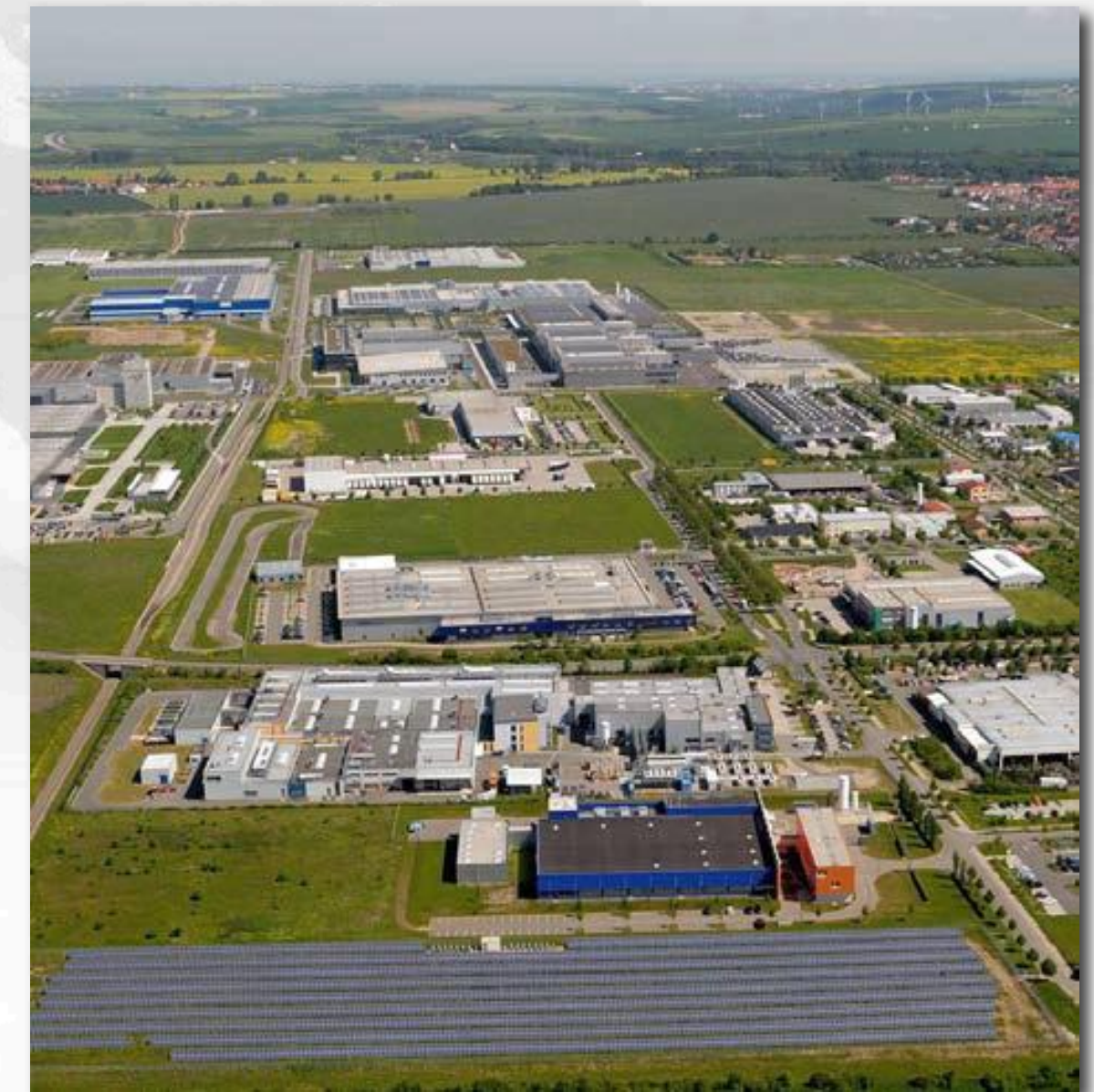
Potential demo plant site, Germany.
