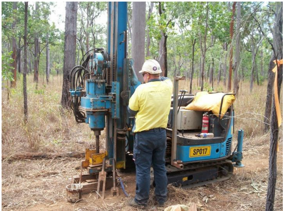
Photo 2: Photo of the rig in operation
