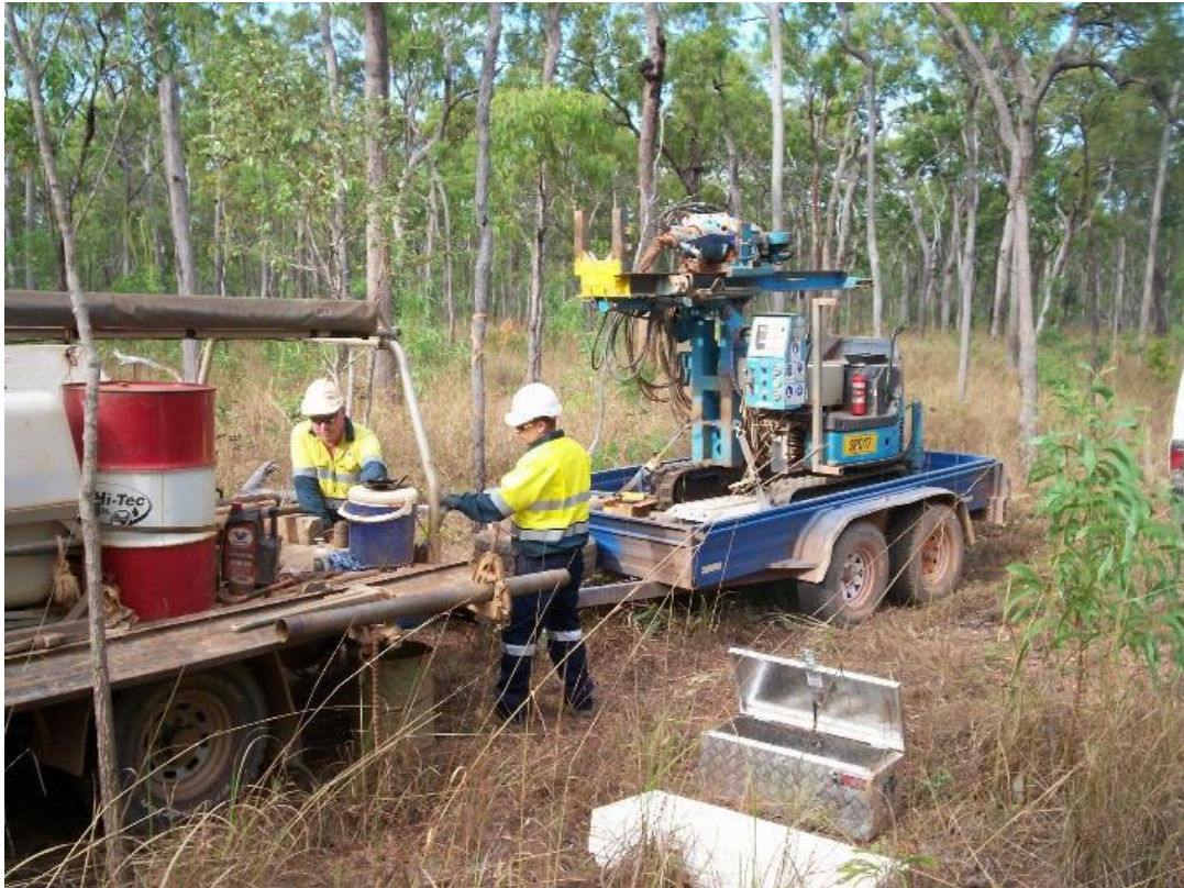
Photo 1: Photo of the sonic drill rig set up
