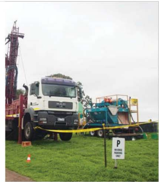
No sumps – closed loop system
