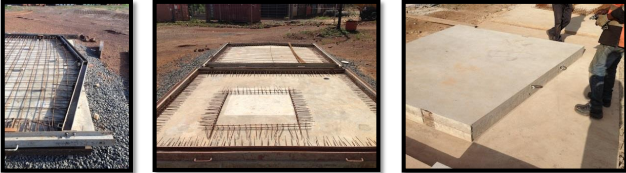
Picture 1: Banfora Gold Project | Newly Engineered Panels for Proposed Resettlement Houses
