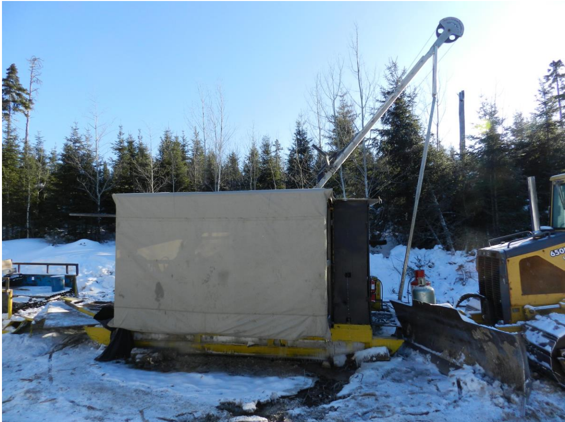
Figure 3: Rig drilling MG-03
