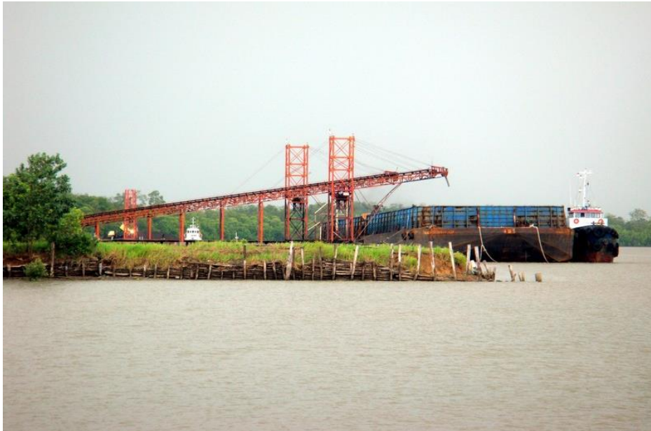
Figure 1: Coal loading facility at Batulicin *
