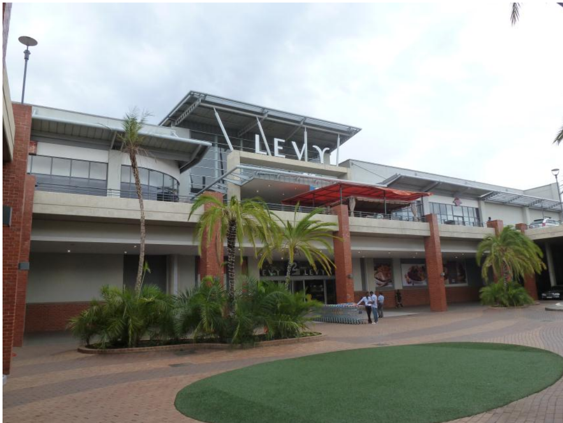
Figure 4: A new shopping mall in Lusaka completed just six months ago. Chronic infrastructure needs are predicted to grow Zambia's cement demand in the decades to come.
