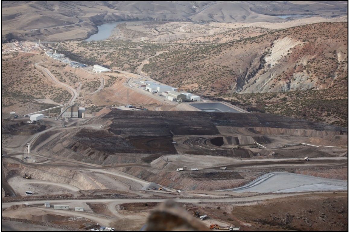
Figure 20-7 Site View from the Project Area – 2
