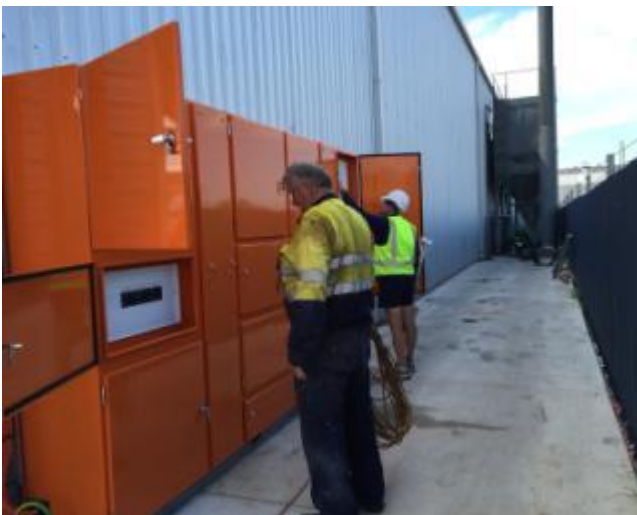
Image 4: 800AMP capacity switchboard connected.
