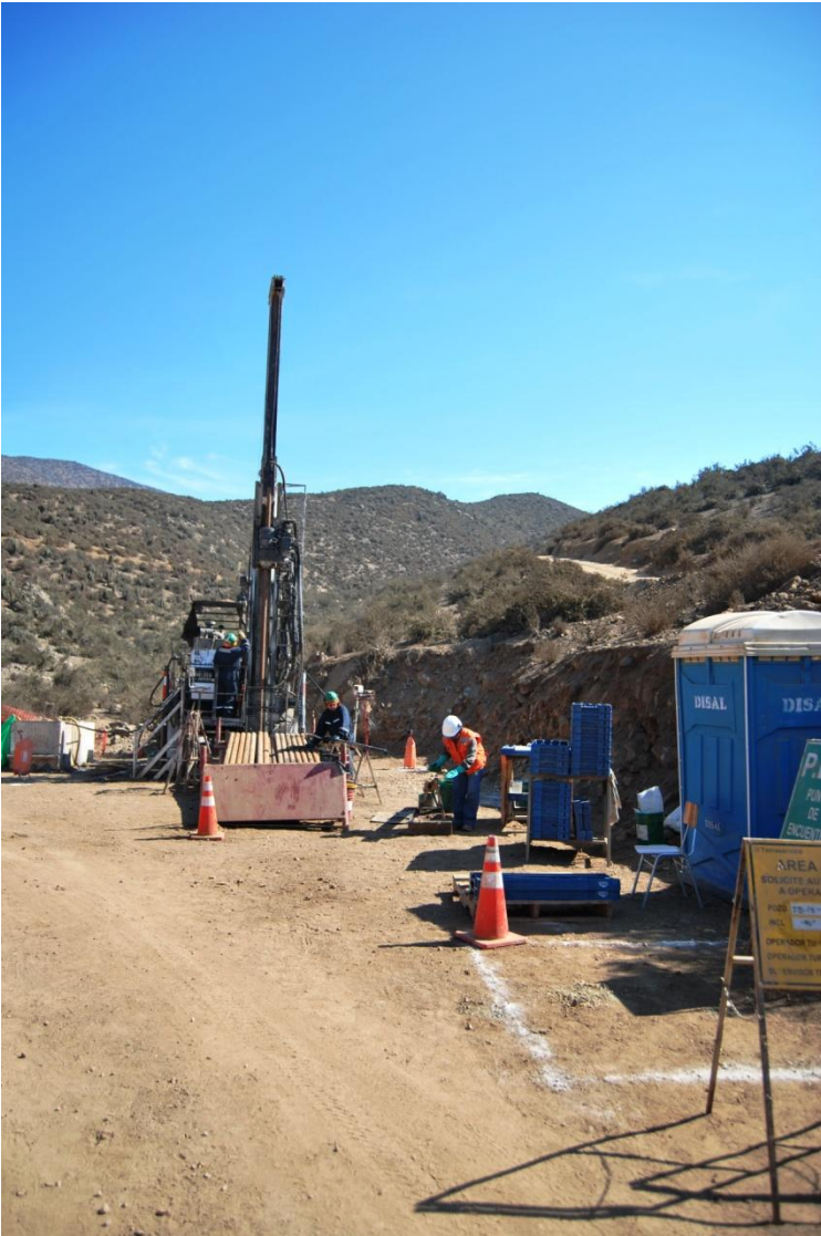
Figure 3: Drilling rig at the Juan Soldado Project
