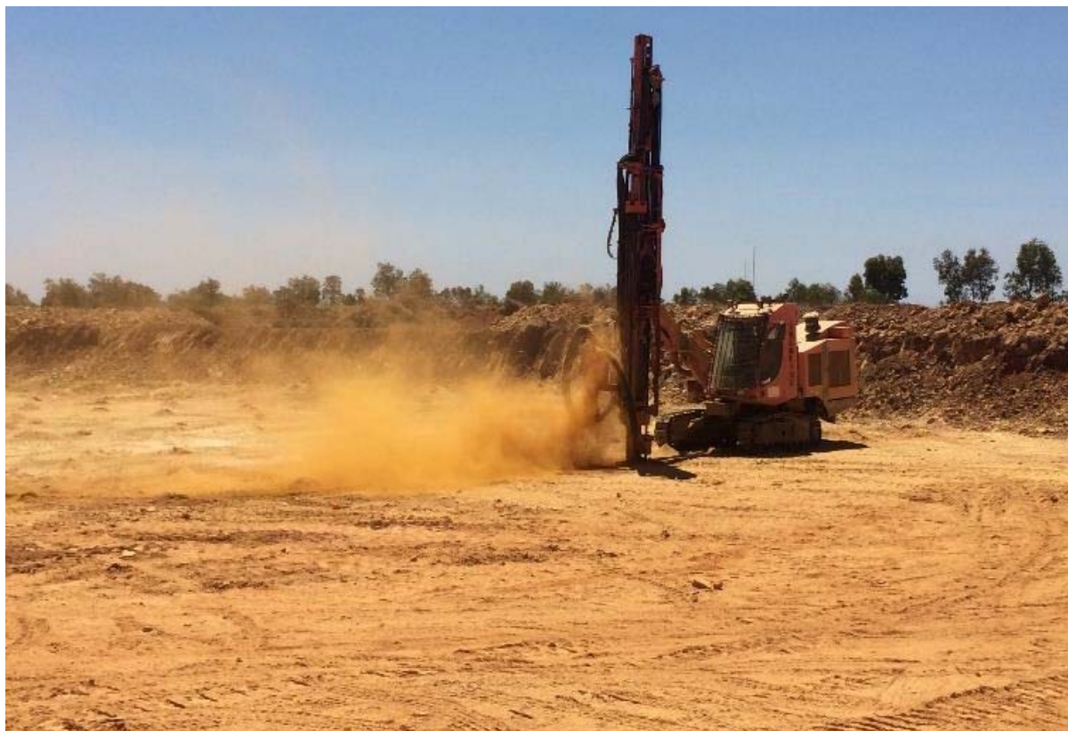
Figure 2. Blast hole drilling at Golden Hind
