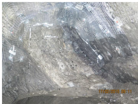
911 narrow vein ore drive with a face grade of 5.6% Ni
