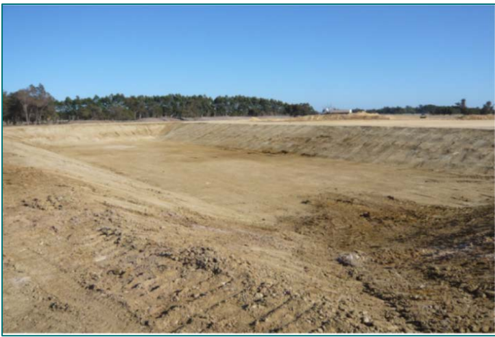
Figure 3: Process water dams being prepared
