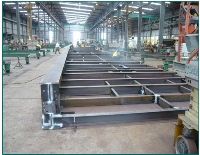
Figure 8: Steel fabrication for the wet concentrator plant
