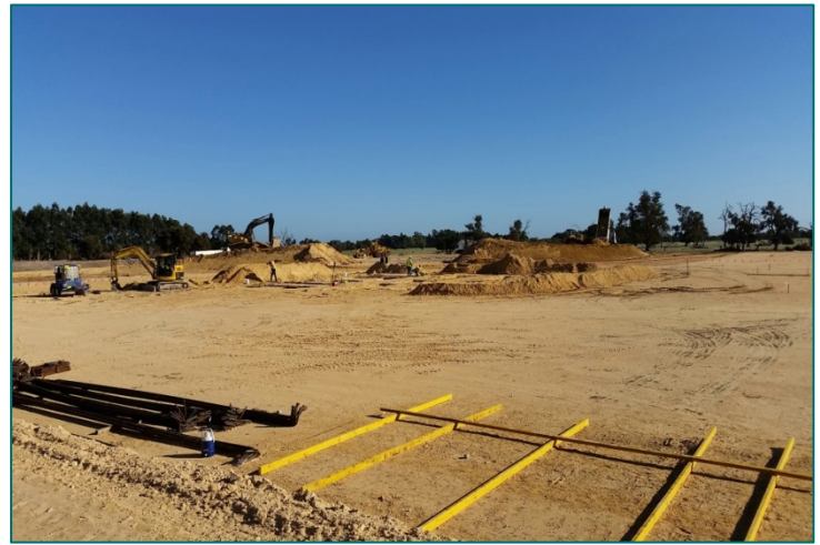
Figure 2: Site works for the wet plant concentrator at Keysbrook
