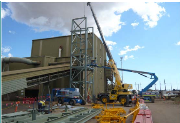
Figure 5: Steel erection at the MSP
