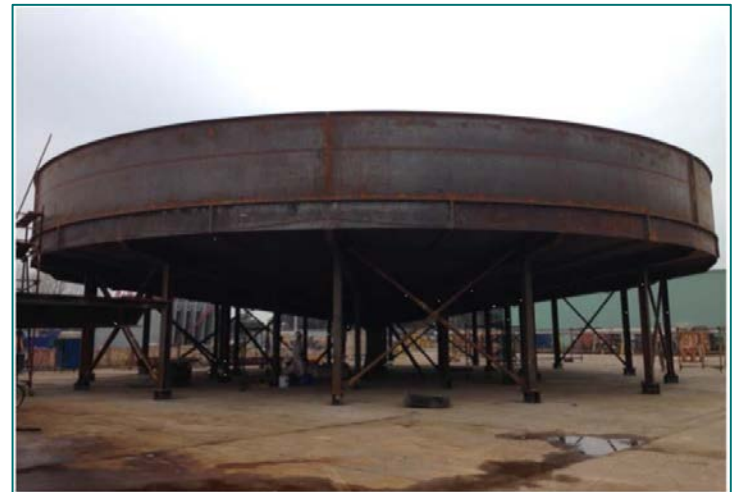
Figure 4: Trial assembly of the thickener
