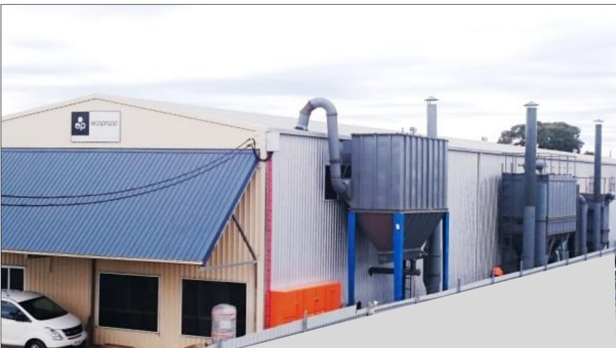
Image 4: The Pilot Plant facility showing External Baghouses completed.
