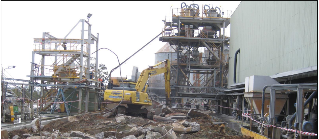
Removal of existing concrete footings for the new CIL plant
