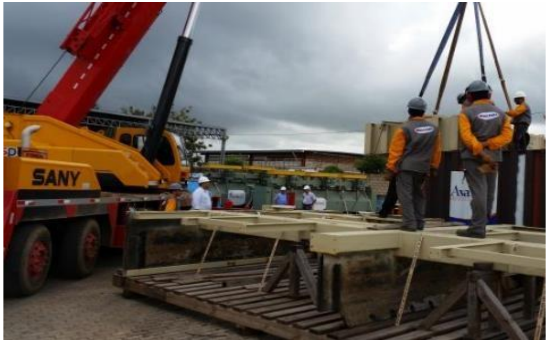
Assembly of an OK 38 Trough Type Flotation Cell
