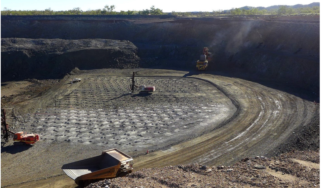
Figure 11: Top image shows the LM2 Pit progressing around the earlier LM1 Pit, which finished at RL152.5. The LM2 Pit has reached RL187.5. Bottom image shows blast-hole drilling at the north-end of the LM2 Pit - the highly weathered supergene ore stands out against the lighter coloured adjacent fresh rock.
