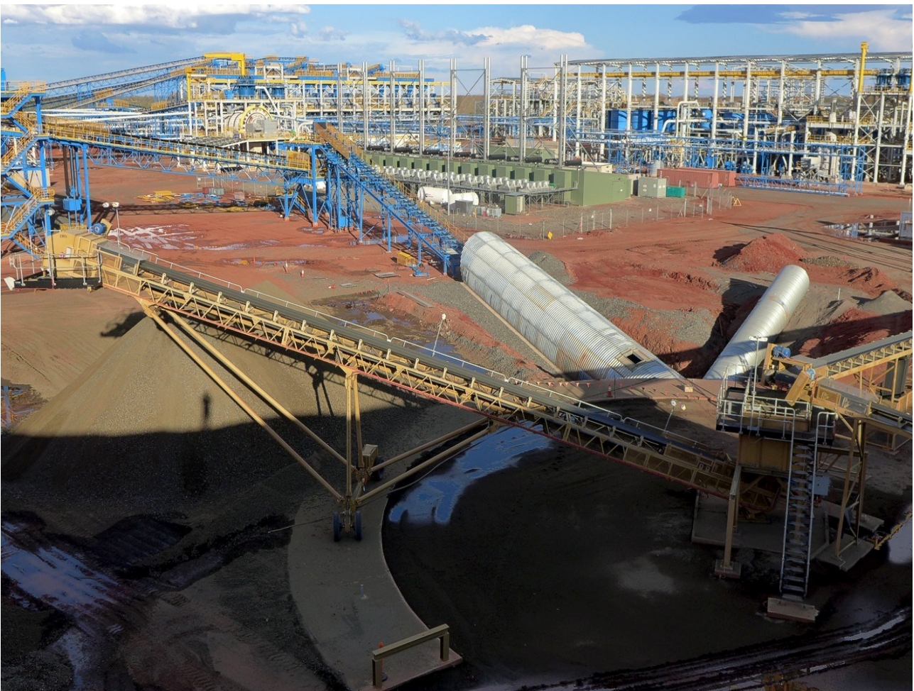
Figure 7: The Process Plant is nearing its final configuration in the foreground is the crushed ore stockpile reclaim tunnel.
