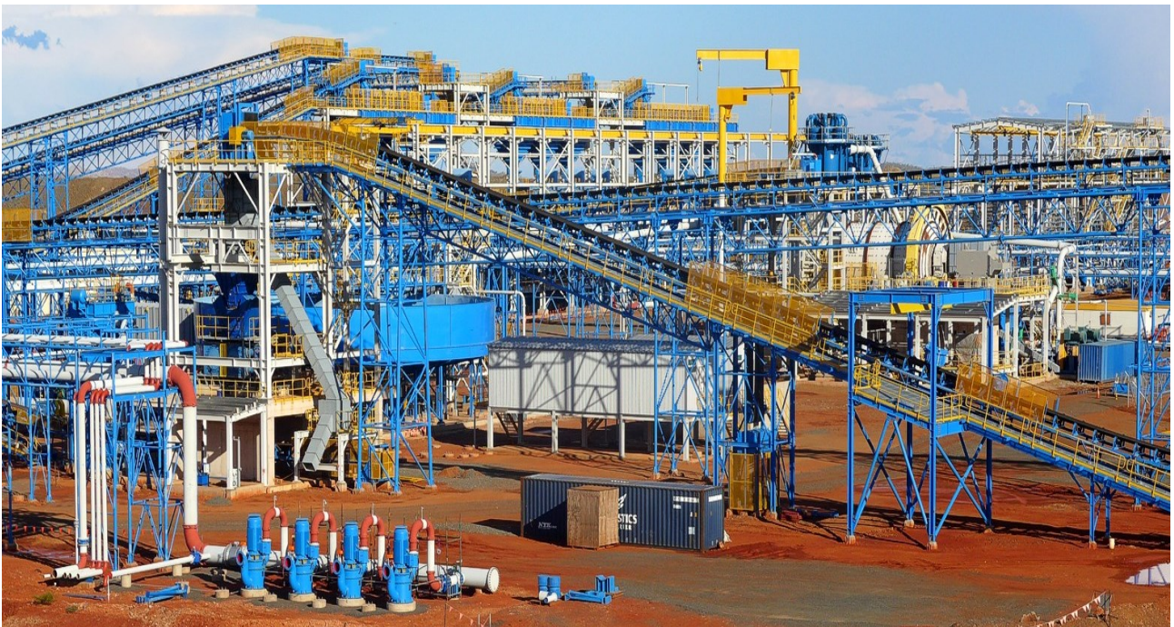
Figure 8: The Process Plant is nearing its final configuration.
