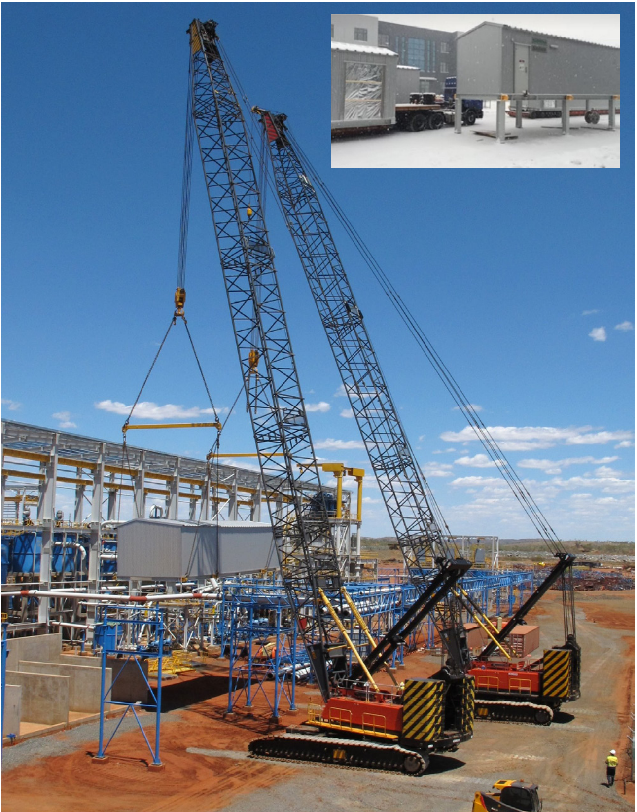
Figure 3: E-houses being lifted into place at Rocklands in 44 degree Celsius heat, after leaving China in sub-zero temperatures (inset).
