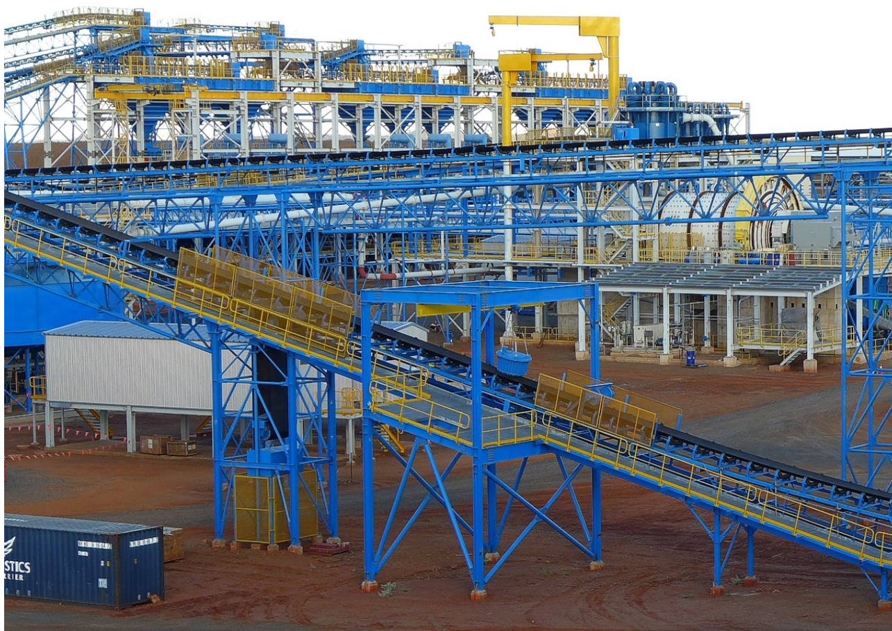
Figure 25: Rocklands Process Plant - installation of electrical cabling has commenced
