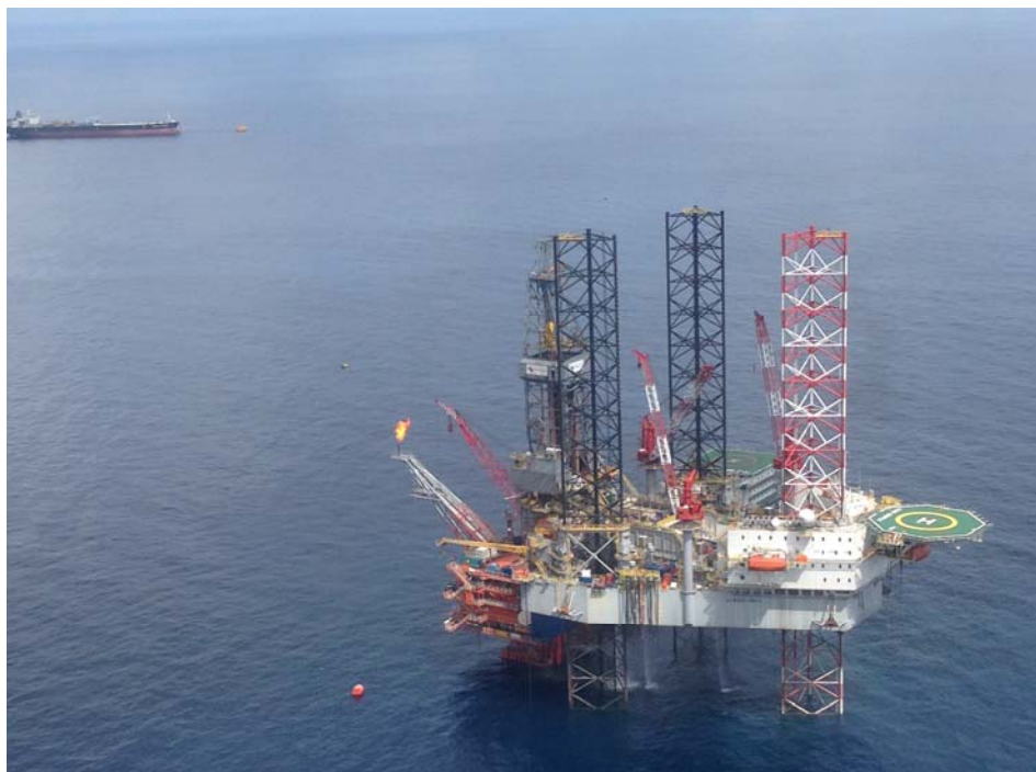
Platform with Manora Princess FPSO in background
