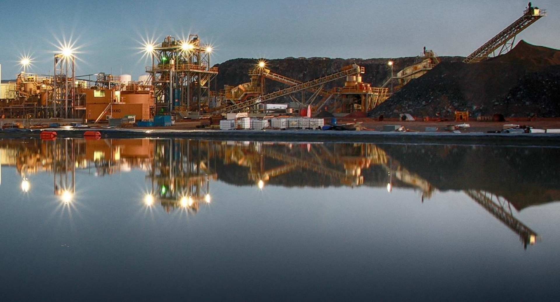
Hera Process Plant
