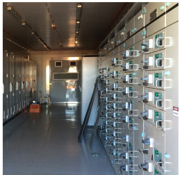
Figure 11 (top to bottom): View of the Process Plant from the ROM, with Crushing Circuit in the foreground, Power Station (recently commissioned) in the middle distance; and each of the 20 E-houses is unique, with purpose built and specific control systems (bottom-left image shows 6,600 Volt Variable Frequency Drives (at Ball Mill) and bottom-right shows Modular Motor Control Centres (Flotation)).
