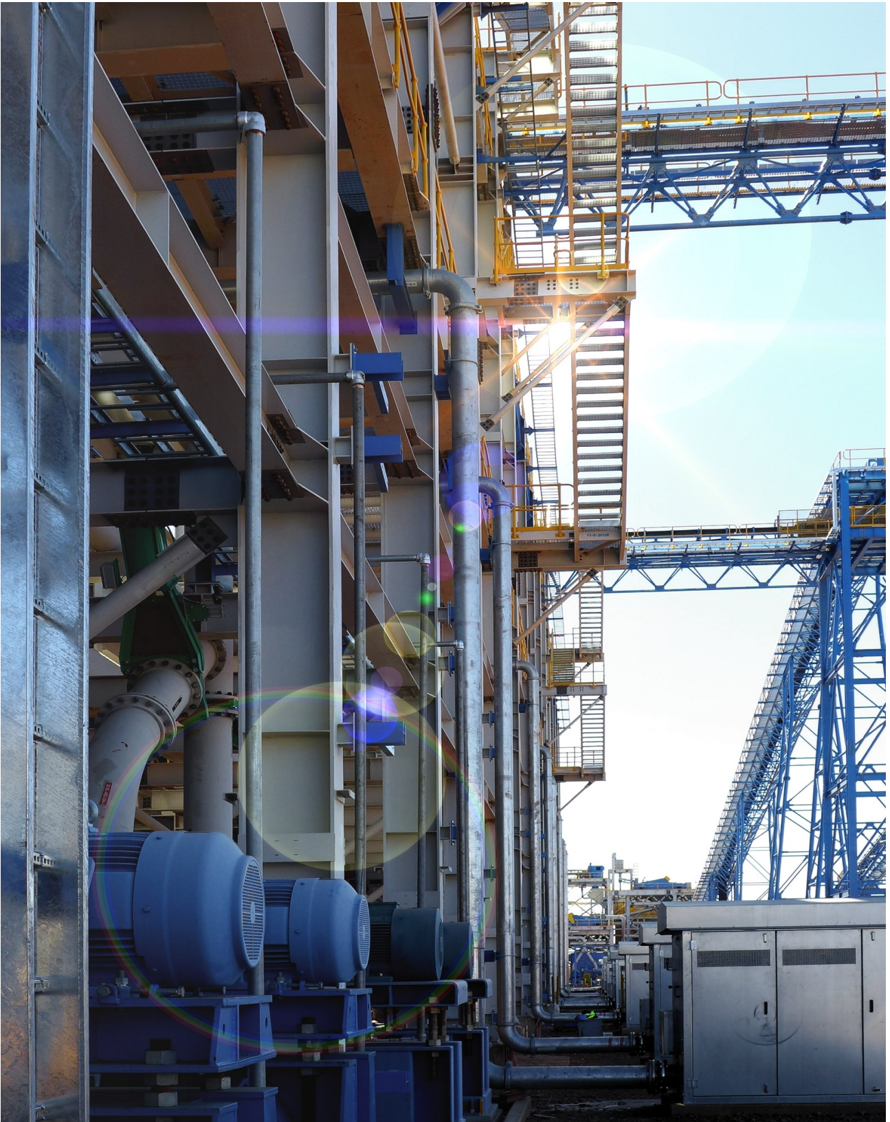
Figure 9: Gravity Jig building
