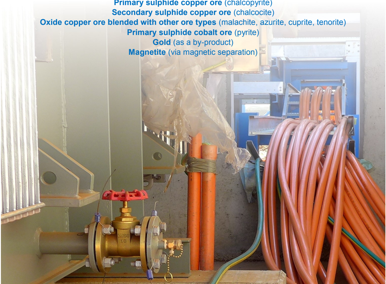
Figure 1: Electrical cable pulled into one of hundreds of termination/connection points across the Project, prior to specialist connection.
