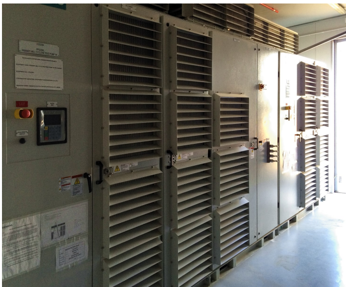
Figure 11 (top to bottom): View of the Process Plant from the ROM, with Crushing Circuit in the foreground, Power Station (recently commissioned) in the middle distance; and each of the 20 E-houses is unique, with purpose built and specific control systems (bottom-left image shows 6,600 Volt Variable Frequency Drives (at Ball Mill) and bottom-right shows Modular Motor Control Centres (Flotation)).
