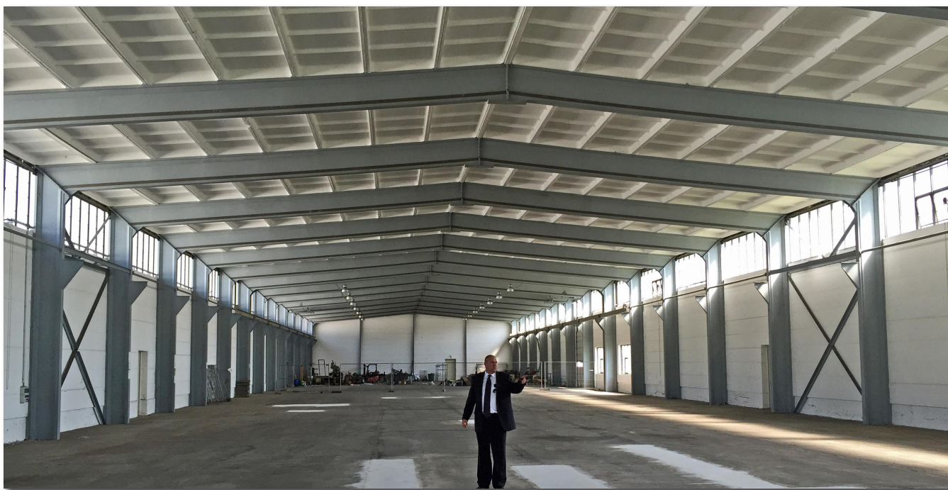
Fig 7 One end of the 1,167m 2 ore dressing/warehouse at Talga's Rudolstadt site, Thuringia, Germany.
