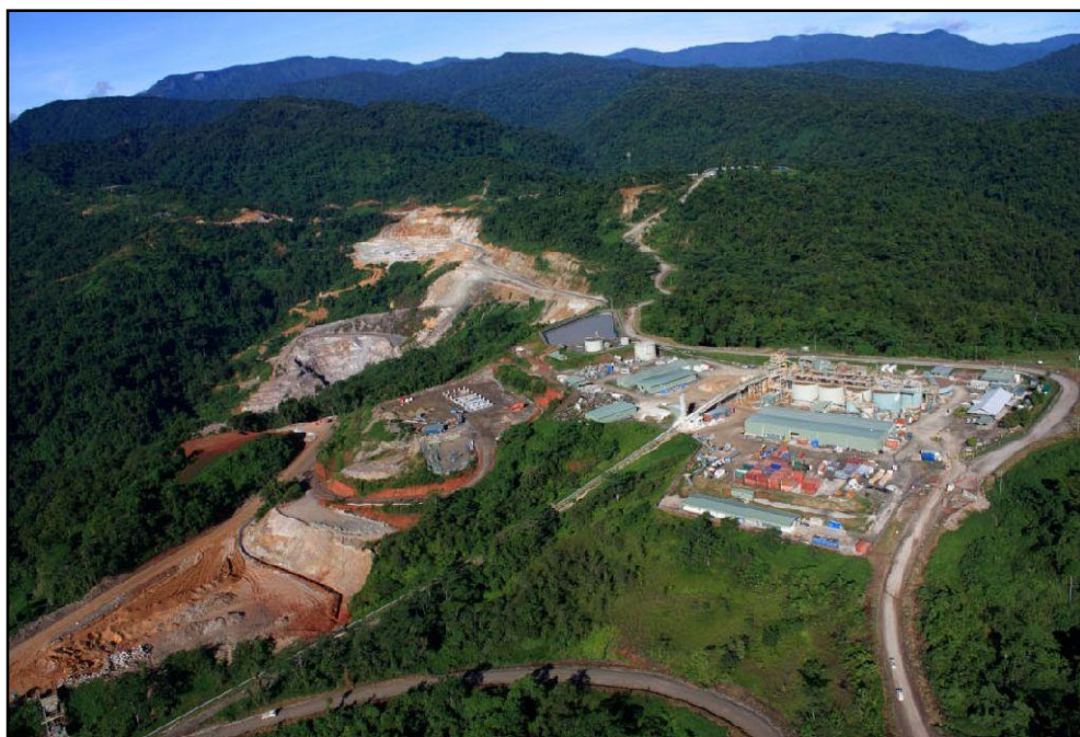
The Gold Ridge Mine processing plant and open pits (St Barbara photo looking south).
