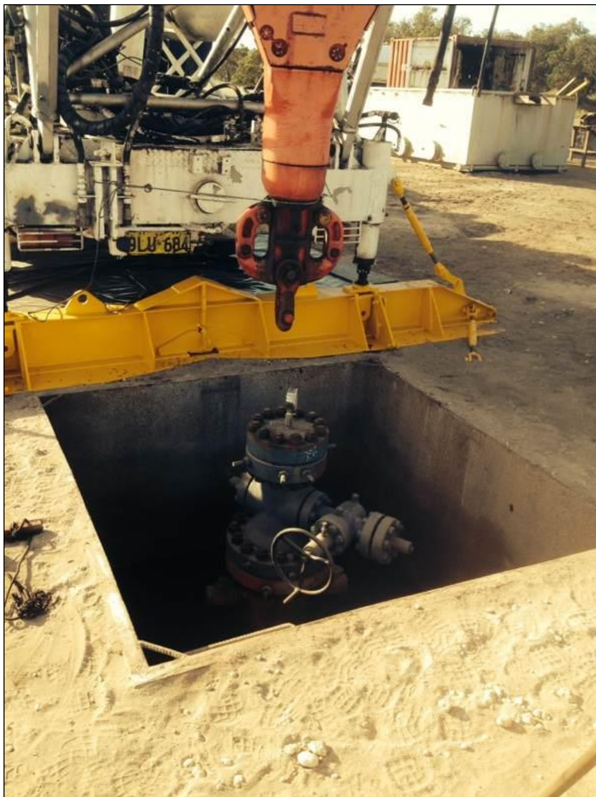
Close up of DCA Rig 6 in close proximity to the B section wellhead inside
