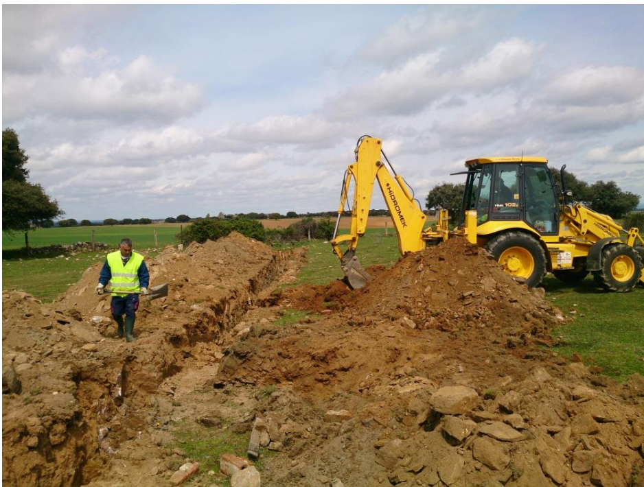
Figure 1: Trenching underway along strike from Toro de Nuevo Banco, Westside Prospect.
