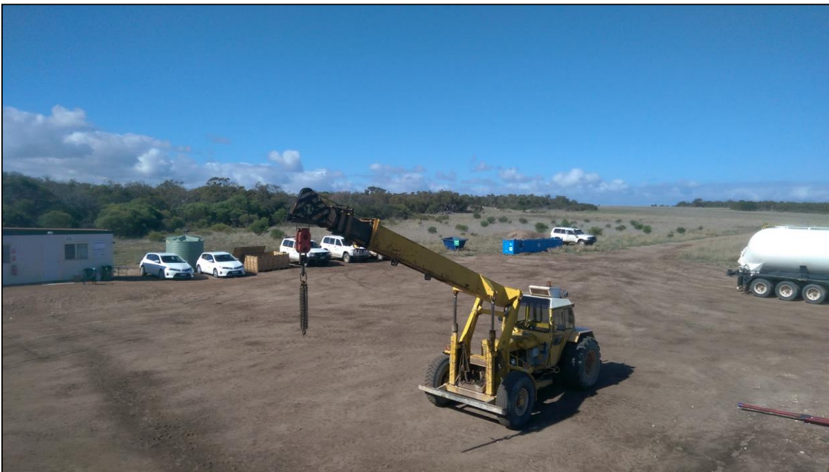
View looking north-west (above) and looking from rig floor south-east
