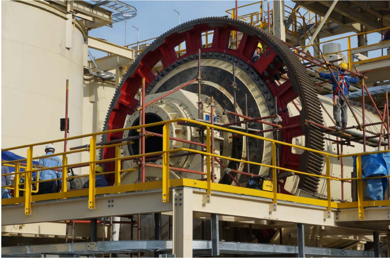
Figure 2. View of both segments of girth installed on the SAG mill
