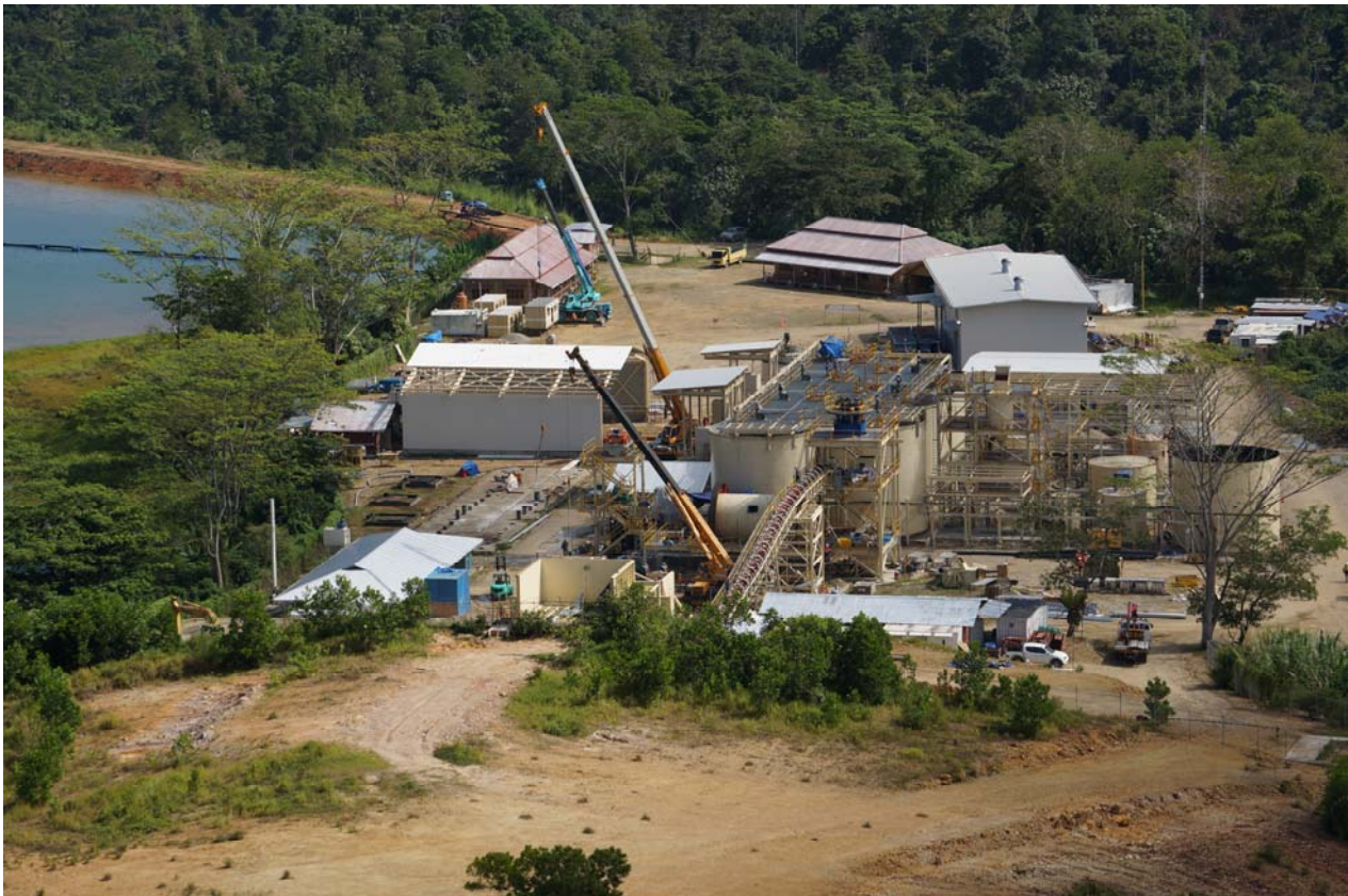
Figure 3. CIL Process Plant and existing tailings storage facility
