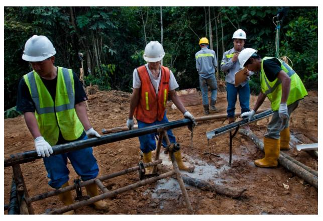
1 - Obtaining coal samples for analysis from core drilling
